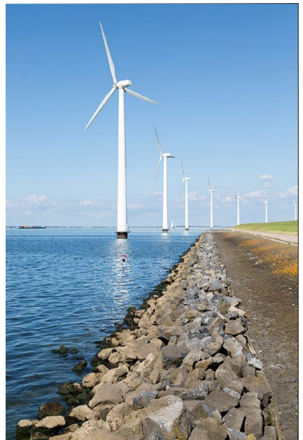
Offshore wind turbines in the Netherlands
